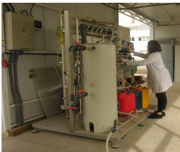
Figure 48. UVC pilot plant installed at PSA facilities.
