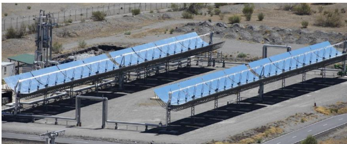
Figure 10. View of the PROMETEO test facility.
