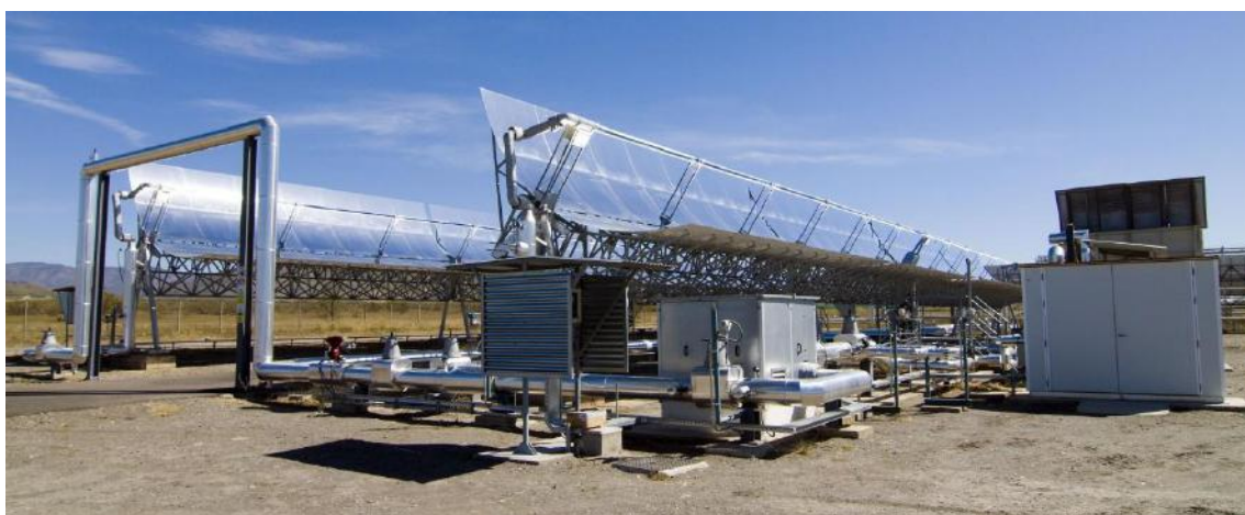
Figure 12. View of the IFL experimental facility (with parabolic troughs) using compressed gas as heat transfer fluid.
