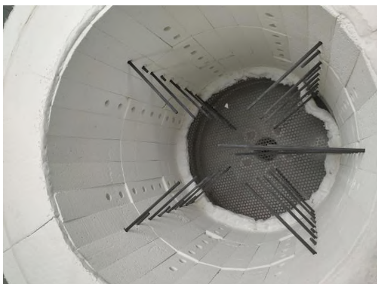
Figure 33. Picture taken from the top of the tank, showing its internal room and thermocouples at different lengths and radial positions.
