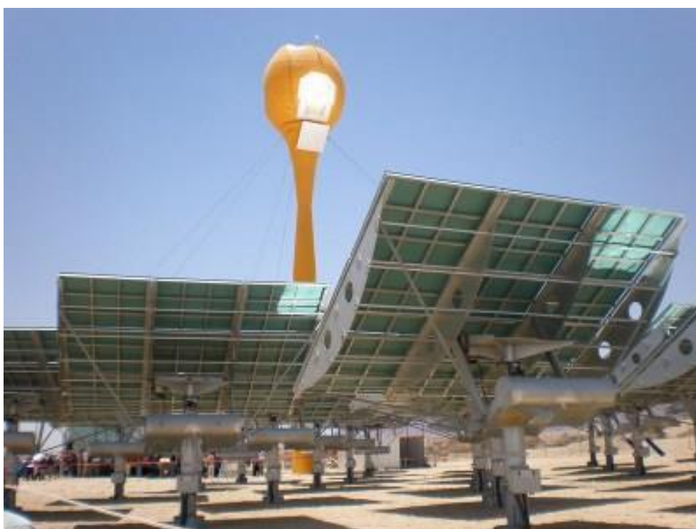
Figure 21. General view of the AORA solar tower facility.
