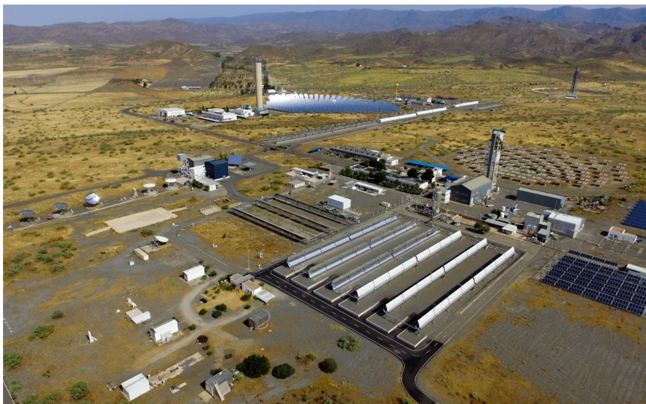
Figure 2. Aerial view of the PSA.
