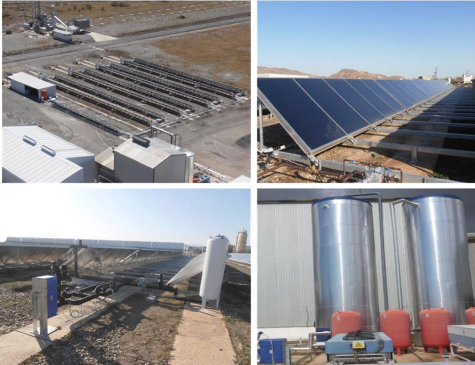
Figure 36. The 606-m 2 large-aperture flat plate solar collector field (AQUASOL-II).
