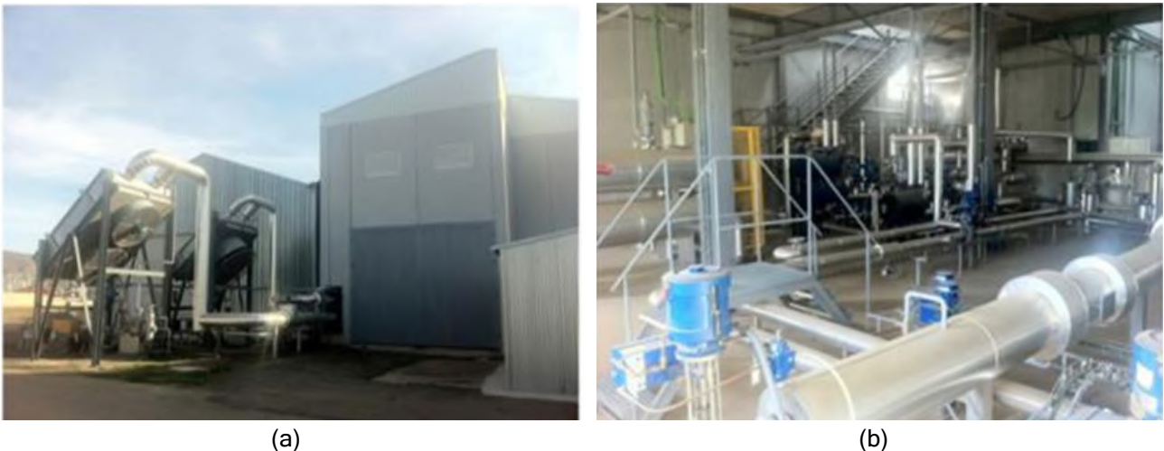
Figure 37. View of the outside of the CSP+D test bed building with the air coolers (a) and partial view of the interior of the CSP+D test bench (b).
