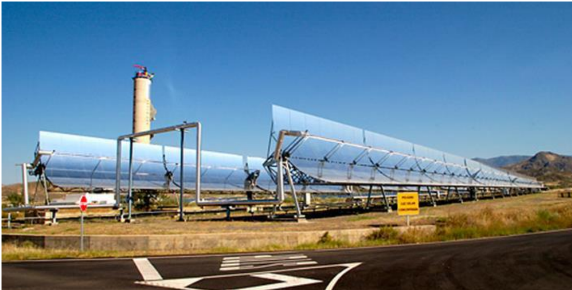
Figure 7. View of the DISC plant solar field in operation.
