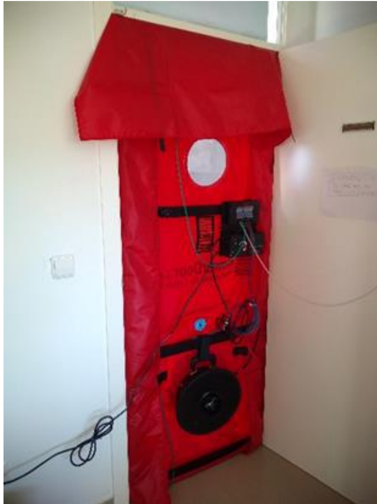
Figure 108. Experiment set up corresponding to a Blower Door Test carried out at the Office Building Prototype at PSA.
