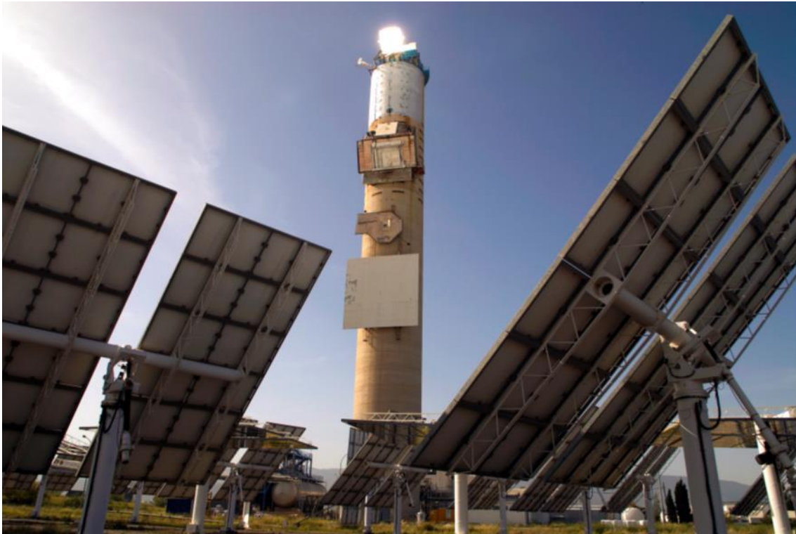
Figure 17. The CESA-I facility seen from the north.
