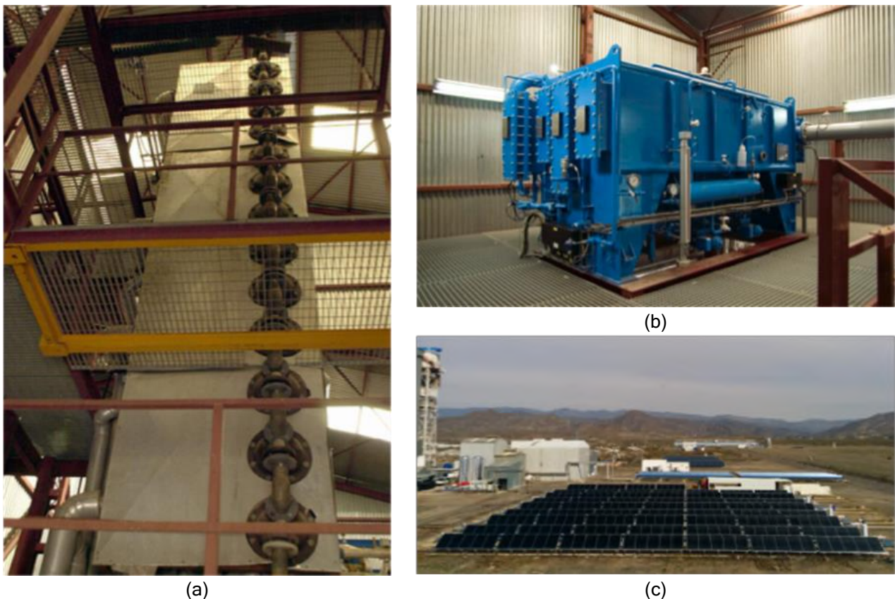
Figure 35. The PSA SOL-14 MED Plant (a) double-effect LiBr-H 2 O absorption heat pump (b) and 606-m 2 flat plate solar collector field (c).
