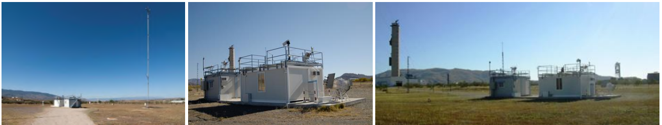
Figure 76. General view of METAS station.
